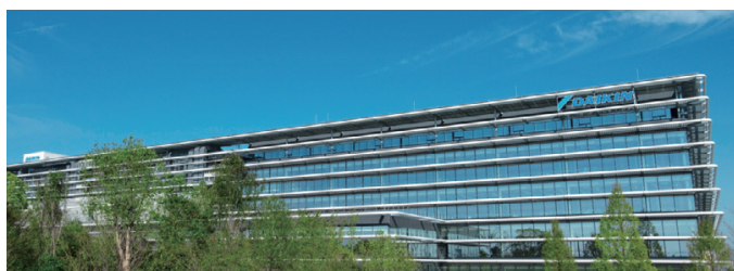
Technology and Innovation Center in Settsu city, Osaka
