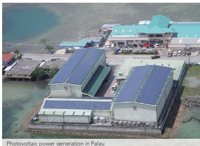
Photovoltaic power generation in Palau
