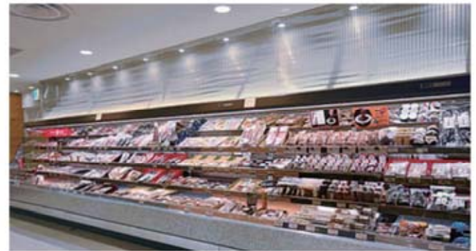
An advanced usage example of a natural refrigerant: refrigeration showcase in Shibuya Hikarie ShinQs. Natural refrigerants are refrigerants that use naturally occurring substances, mainly ammonia, CO 2 , water, air, hydrocarbons, etc., instead of fluorocarbons that have a high greenhouse effect.
