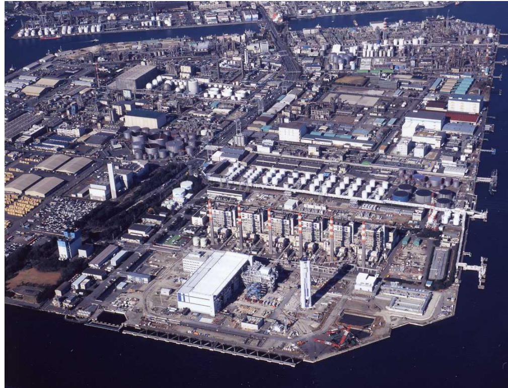
Kawasaki Thermal Power Plant *2
