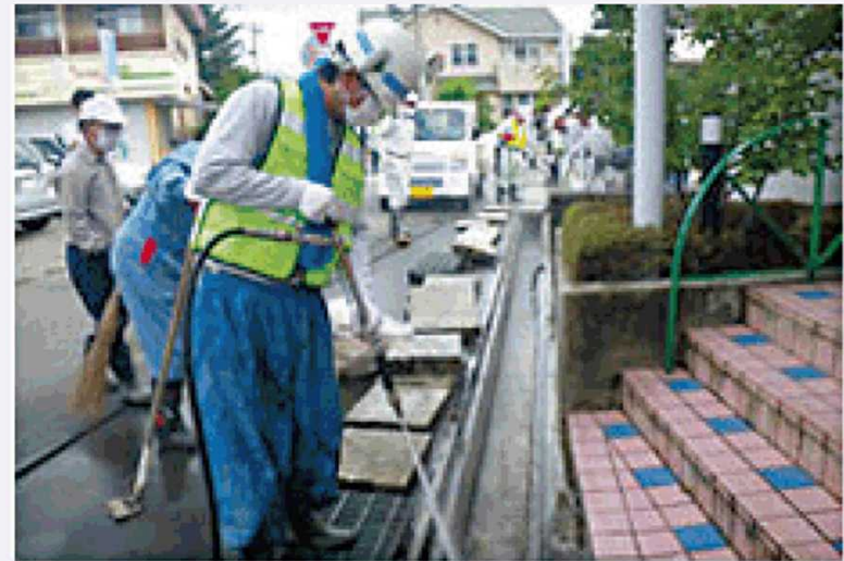
Removing sludge from ditches
