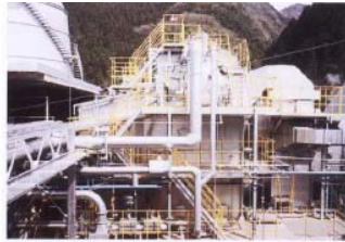
Wood Chip Burning Boiler
