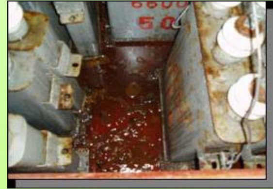
[Improper storage of PCB waste]
