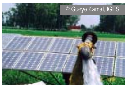
Solar water pumping in Chandigarh, India
