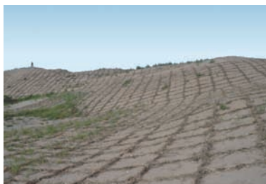
Photo 2 Straw checkerboards
