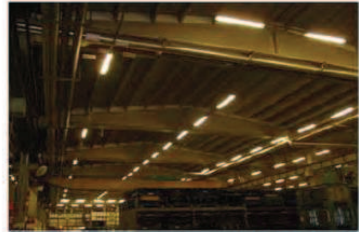
Lamps were changed to energy efficient fluorescent lamps
