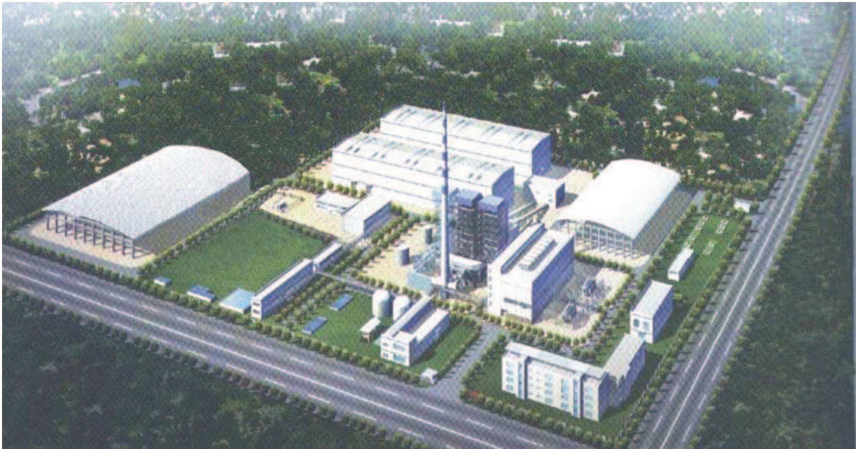
12 MW Biomass Power Plant in Banga, Aklan
