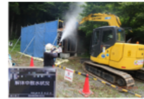
Demolition of a damaged house, etc.
