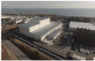
Temporary Incineration Facility in Okuma Town (December 2017)
