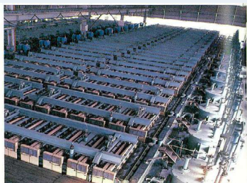
Okayama Chemical Co., Ltd. Electrolytic bath (October, 1970)
