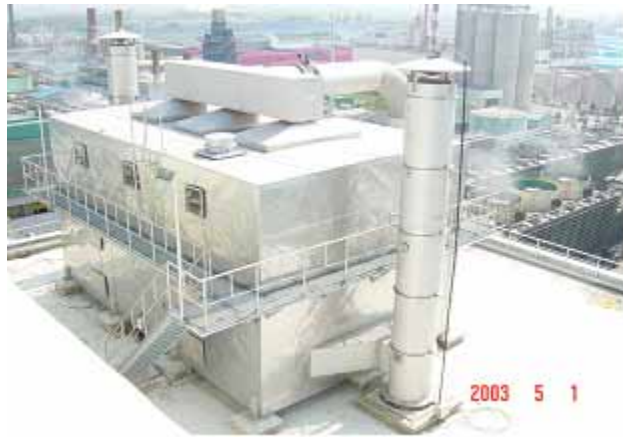
Figure 9. Long view of KAVOTEC biotrickling filter installed at BASF vitamin manufacturing factory
