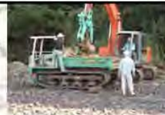
Cleaning by heavy machinery
