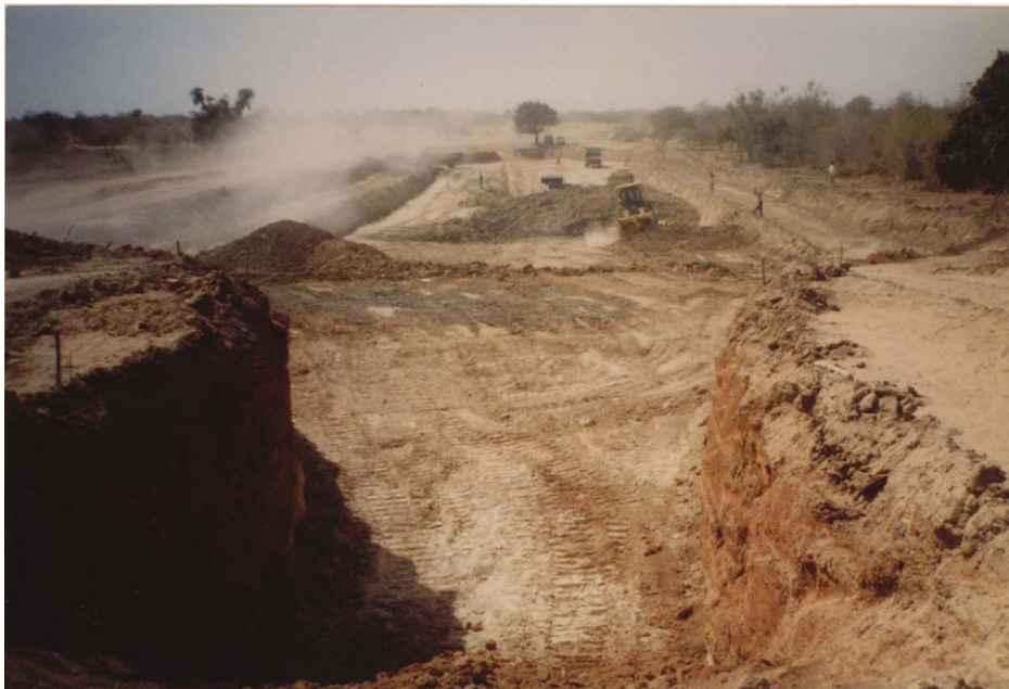
Photo 4.2: Construction of the subsurface dam -2
