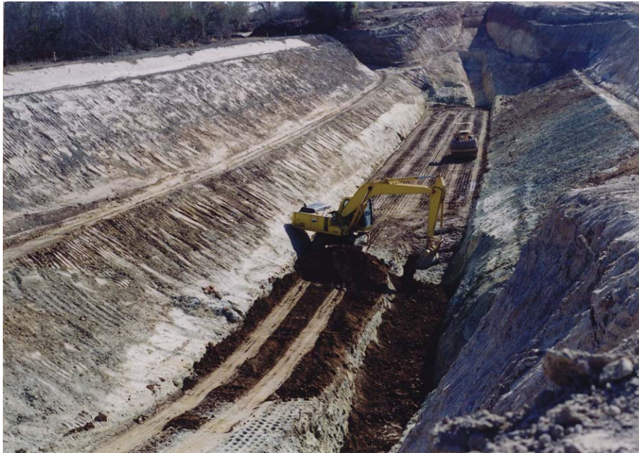
Photo 4.3: Construction of the subsurface dam -3
