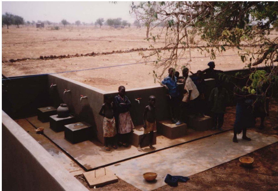
Photo 7.3: Water-supply station for domestic use, installed in Kombangbedo Village
