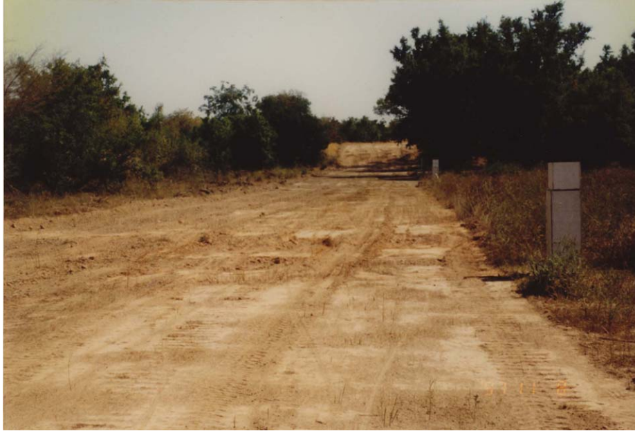
Photo 4.1: Construction of the subsurface dam -1
