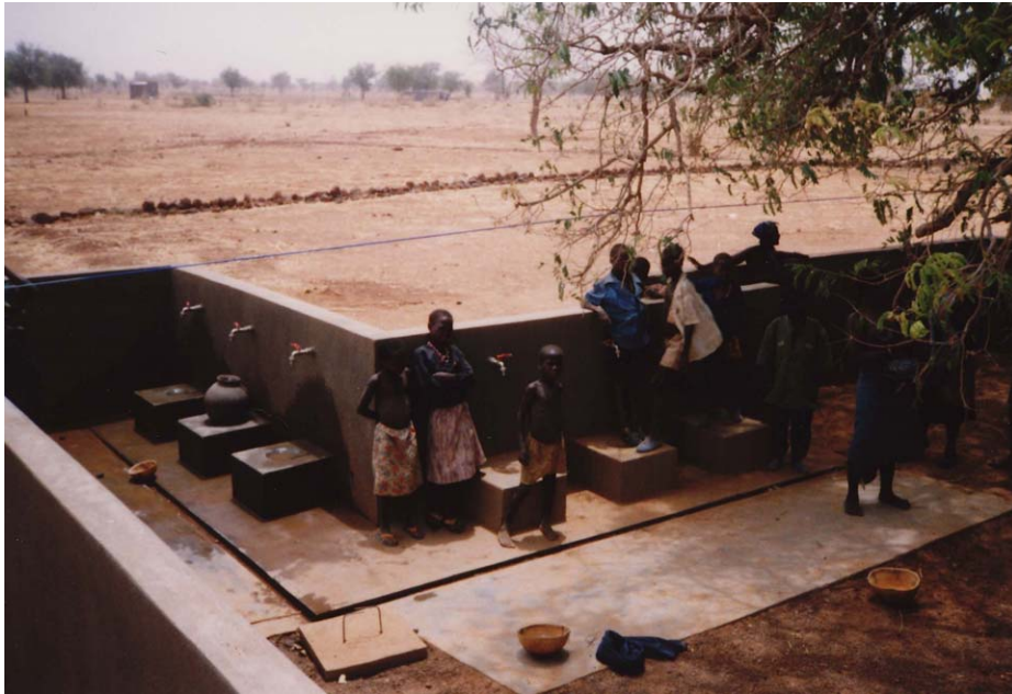
Photo 7.3: Water-supply station for domestic use, installed in Kombangbedo Village
