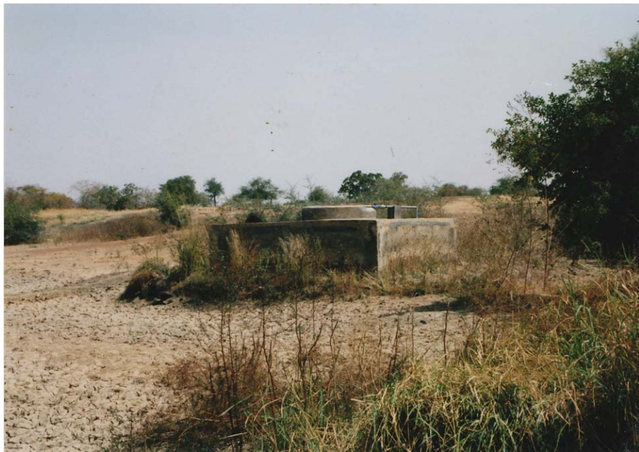
Photo 7.2: Pumping well installed in the reservoir area of the subsurface dam (The well is surrounded by concrete walls for protection from river floods.)
