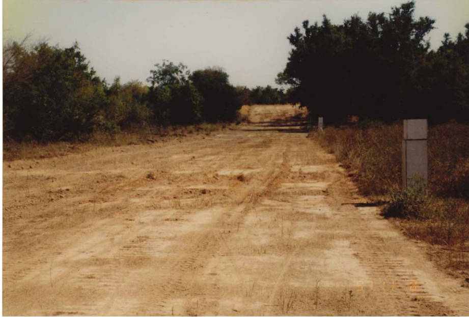
Photo 4.1: Construction of the subsurface dam -1
