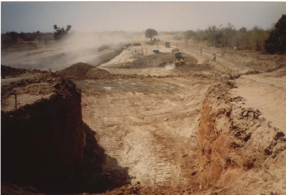
Photo 4.2: Construction of the subsurface dam -2
