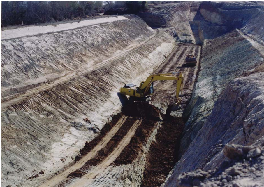
Photo 4.3: Construction of the subsurface dam -3
