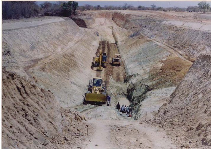
Photo: Construction of the subsurface dam
