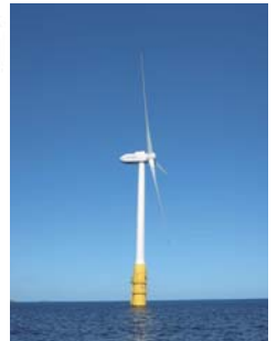
Floating Wind Turbine Facility
