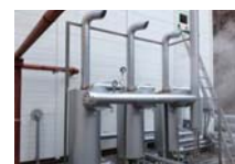
Heat exchanger for collecting untouched vapor heat
