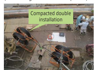
high speed construction system (shortening of construction period)
