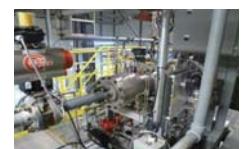
Permanent-magnet and high-speed turbine generator for ammonia rated at 87 kW with an average turbine efficiency of 77.4%
