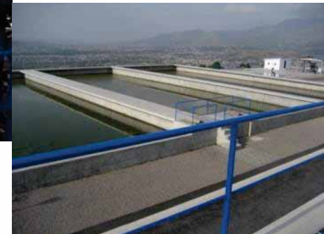
Water supply facility (Pakistan)
