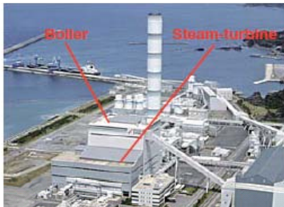
Misumi coal-fired power plant 1000 MW, 24.5 MPa \times 600 ^{\circ} C/600 ^{\circ} C operation started in 1998
