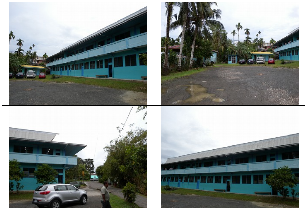
図 2.3-14 現地調査写真 (Maris Stella Elementary School (Lower campus) )
