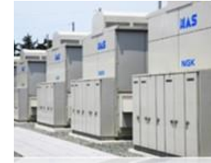
Large Capacity Secondary Battery
