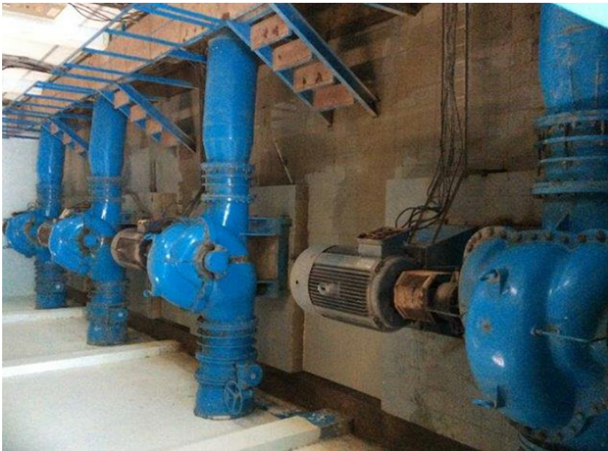
LOW LIFT pump house
