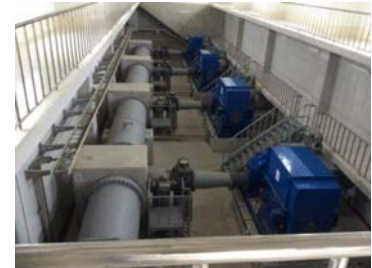
Pump room in Nyaung Hnit Pin
