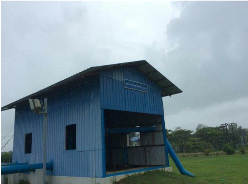
Back Wash Pump Station
