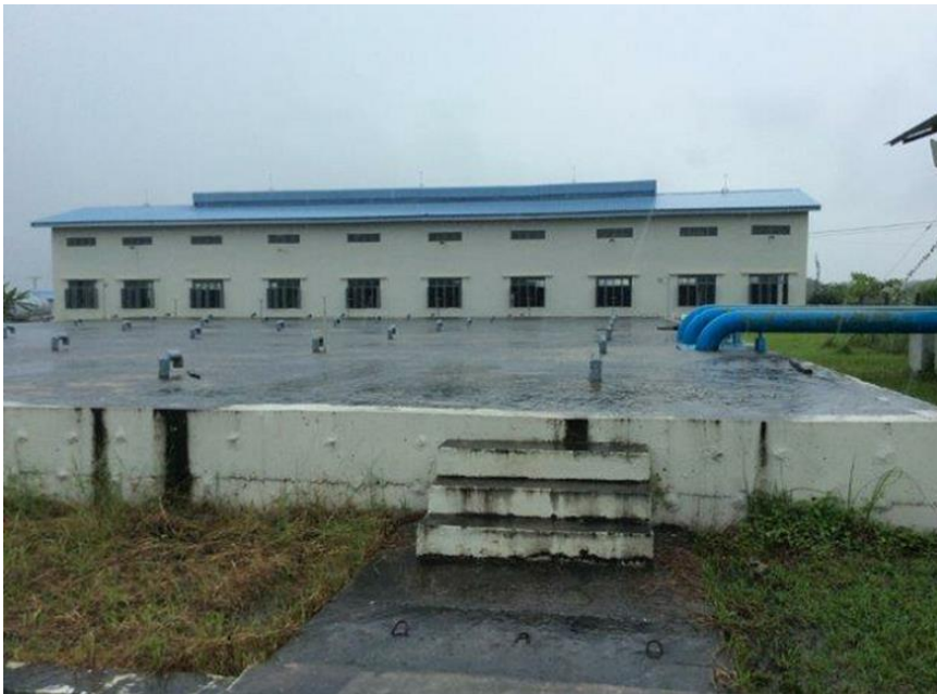
treated water reservoir
