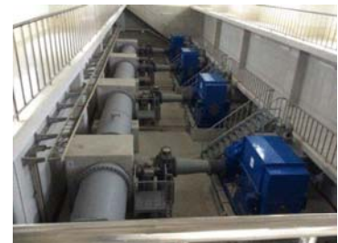
Pump room in Nyaung Hnit Pin
