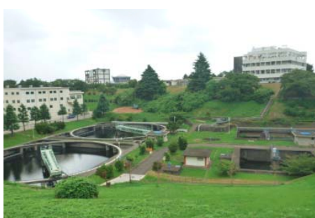
Overall View of Nagasawa
