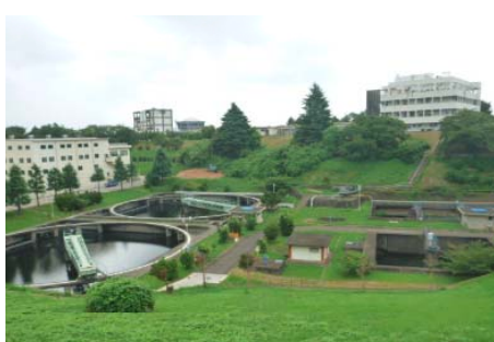
Overall View of Nagasawa
