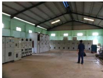
Electric room (PV – related equipment can be stored) in Nyaung Hnit Pin
