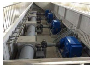
Pump room in Nyaung Hnit Pin
