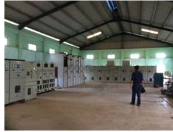
Electric room (PV – related equipment can be stored) in Nyaung Hnit Pin
