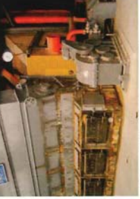
• 25 Ton coal boiler for China government department
