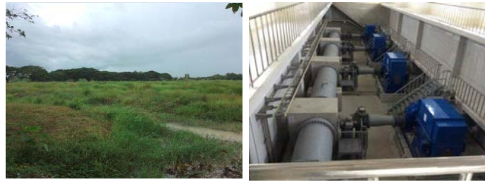
PV site and Pump room in Nyaung Hnit Pin
