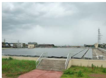
PV modules installed above reservoir
