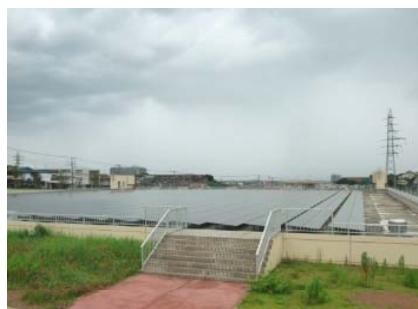
PV modules installed above reservoir
