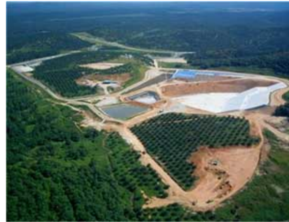
Sanitary landfill project at Bukit Tagar
