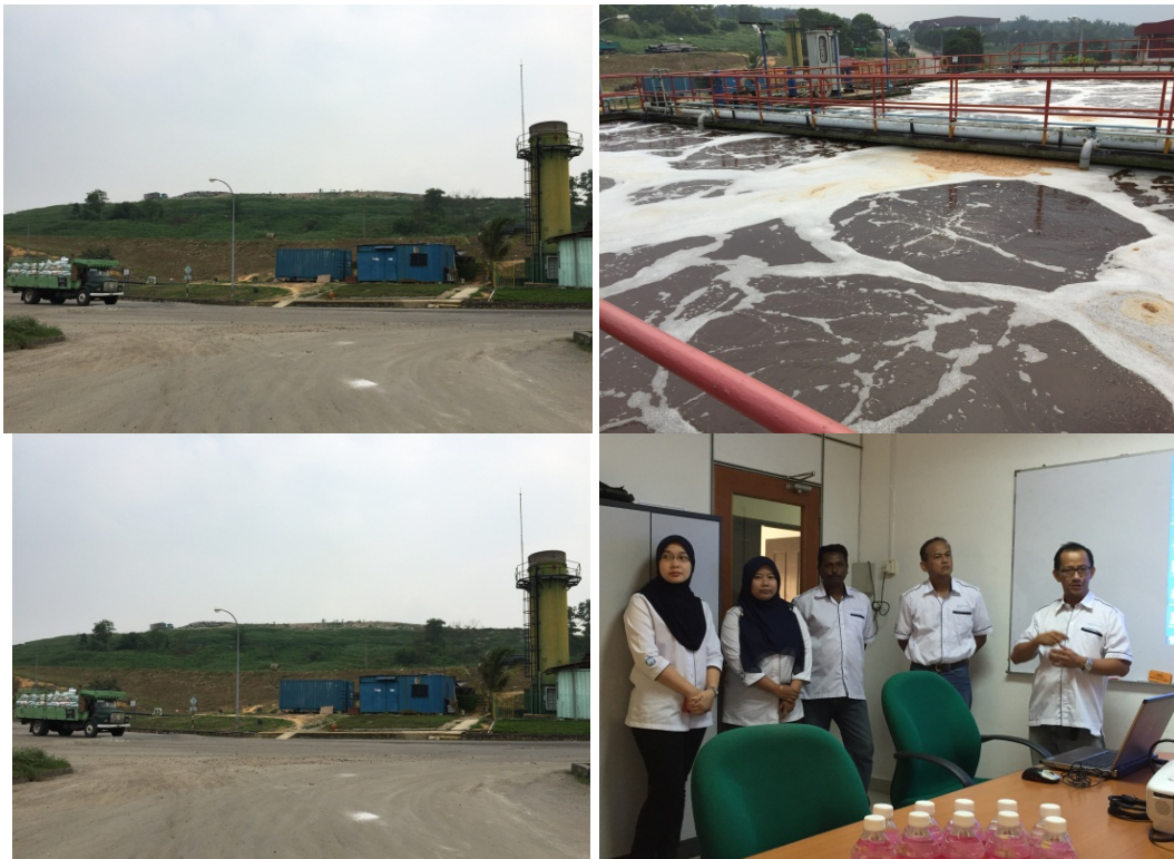
Photos of Seelong Landfill
