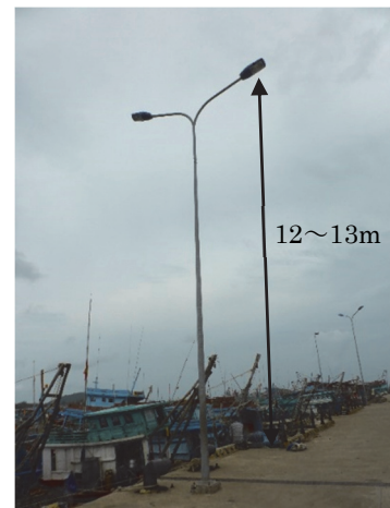
Photo 4.2.1.1 Lighting facilities of An Thoi Harbour
