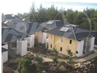
Figure 4.4.1.4 Solar water heater installed at Eden Resort on Phu Quoc Island (manufactured by SolarBK)
