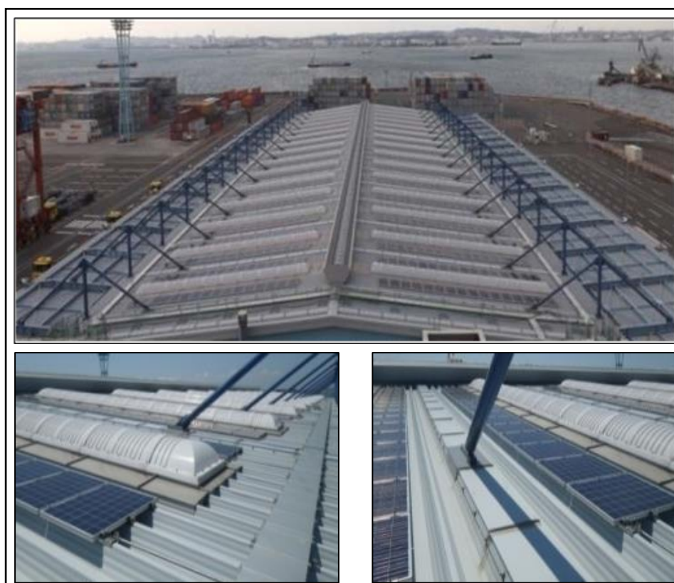
Figure 63 PV Panels on CFS Roof with Barrel-vaulted Skylight Windows at Minami Honmoku Pier of Yokohama Port
