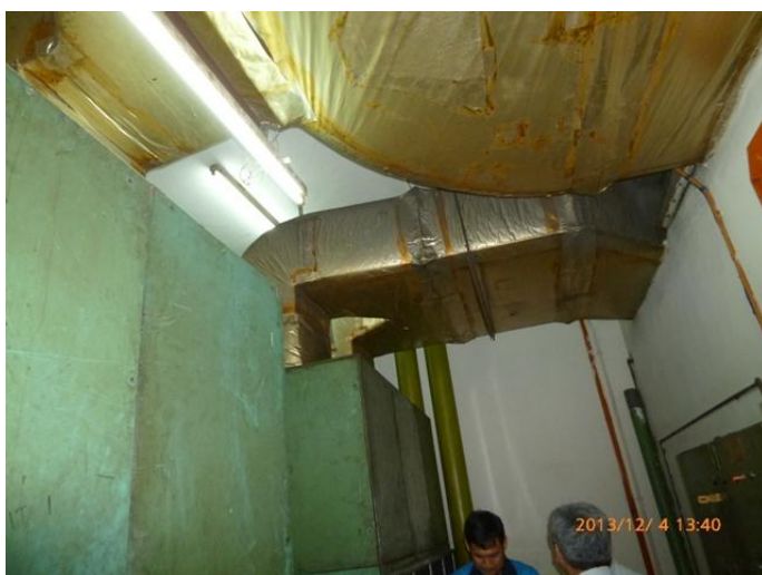
Photo 3-3-9 A supply duct in an air-cooled package has no damper installed on it for controlling the airflow.
