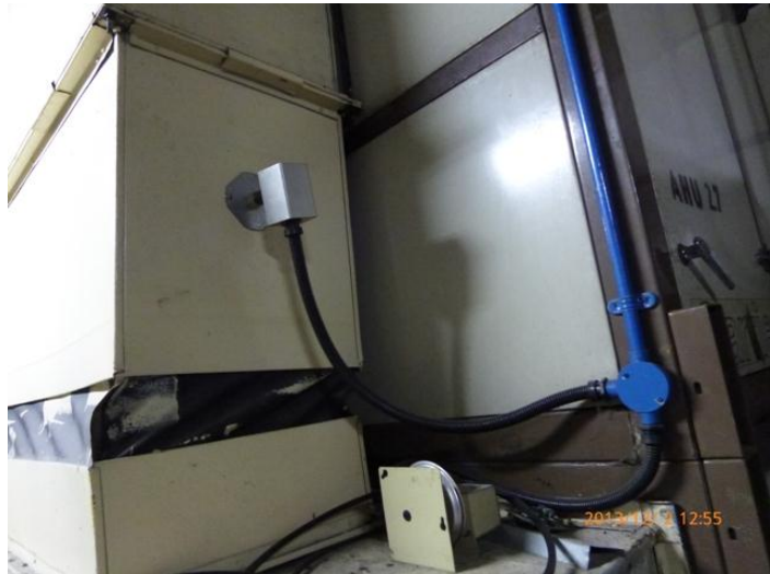
Photo 3-3-20 An AHU supply duct equipped with a temperature sensor for an automatic two-way valve for controlling the chilled water flow rate.
