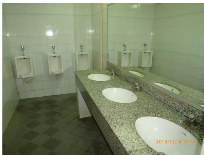
Photo 3-3-11 The toilet stalls and urinals are equipped with a flush valve. Water saving is possible by replacing the valves with automatic washing system.
