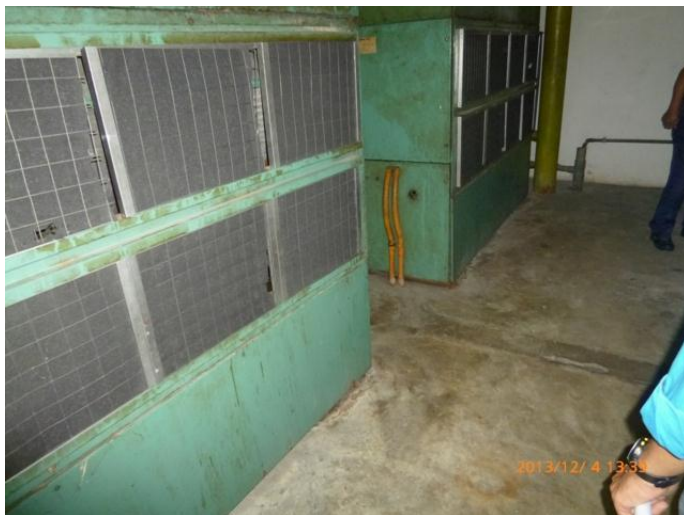
Photo 3-3-8 The filters in an air-cooled package are kept clean.
