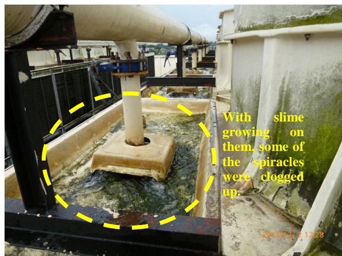
Photo 3-3-16 Distribution basin on the cooling tower
