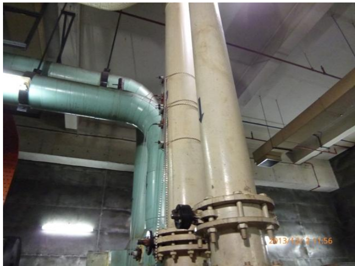
Photo 3-3-18 An ultrasonic flow rate sensor installed on a chilled water pipe
