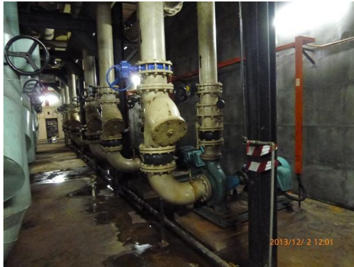
Photo 3-3-15 Cooling water pump left out of energy-saving control
