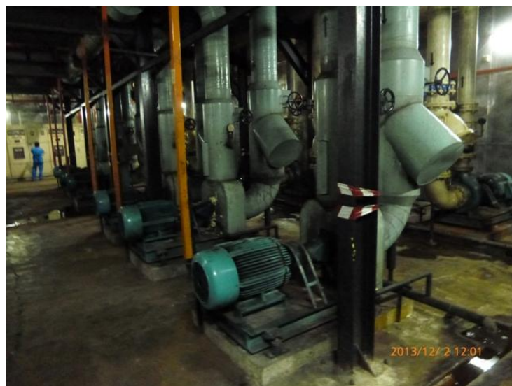
Photo 3-3-14 Chilled water pump left out of energy-saving control
