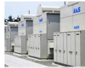
Large Capacity Secondary Battery
