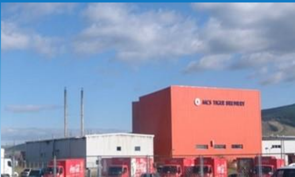
Introduction of Thermal Storage Heater
