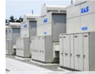
Large Capacity Secondary Battery
