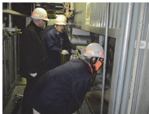
Boiler combustion section (manufactured by Hitachi Zosen Corporation)
