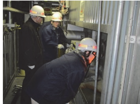
Boiler combustion section (manufactured by Hitachi Zosen Corporation)
