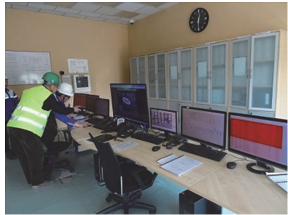
vi) Control room at SWF
