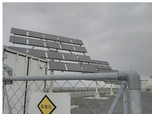
Solar PV facility
