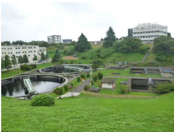
Water purification plant
