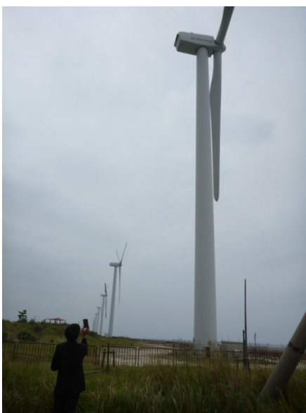
Wind power facility
