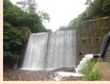
Small hydro power plant utilizes check dams
