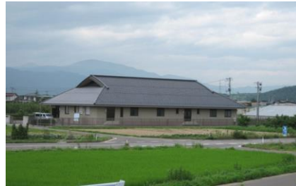
Drainage treatment plant in Yamaguchi District
