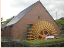
The Village of Four Seasons' small hydro power generation facility leverages local resources and the technologies of a local corporations .
