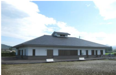
Drainage treatment plant in Oda District
