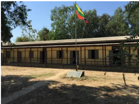
Local elementary school
