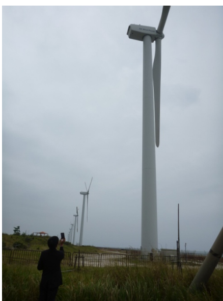
Wind power facility
