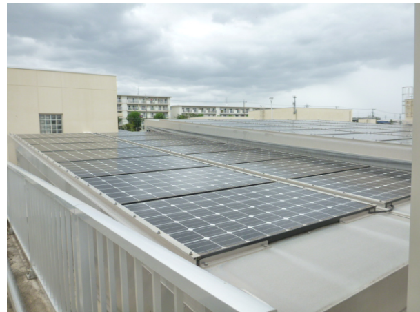
Solar panel introduced on the cover of plant
