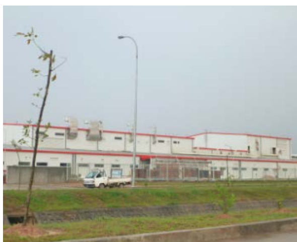
Overview of Food Factory introduced Once-through boiler
