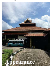
Ferry Terminal Nongsa
