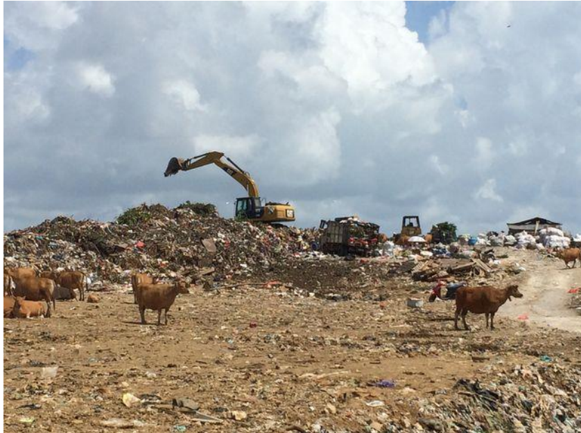
Figure 2.14 Block 1 being used for land reclamation (July 2016)
