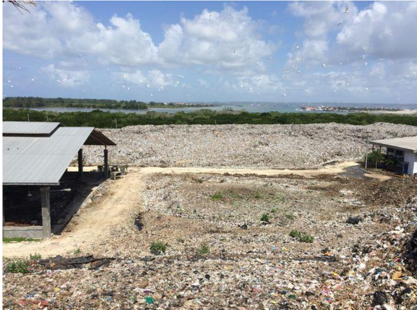
Figure 2.18 July 2016 (the gas engine building on the right side of the photo)
