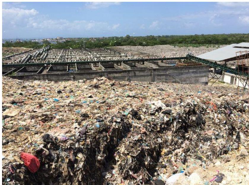
Figure 2.17 NOEI facilities (concrete tanks that look like methane fermentation tanks)
