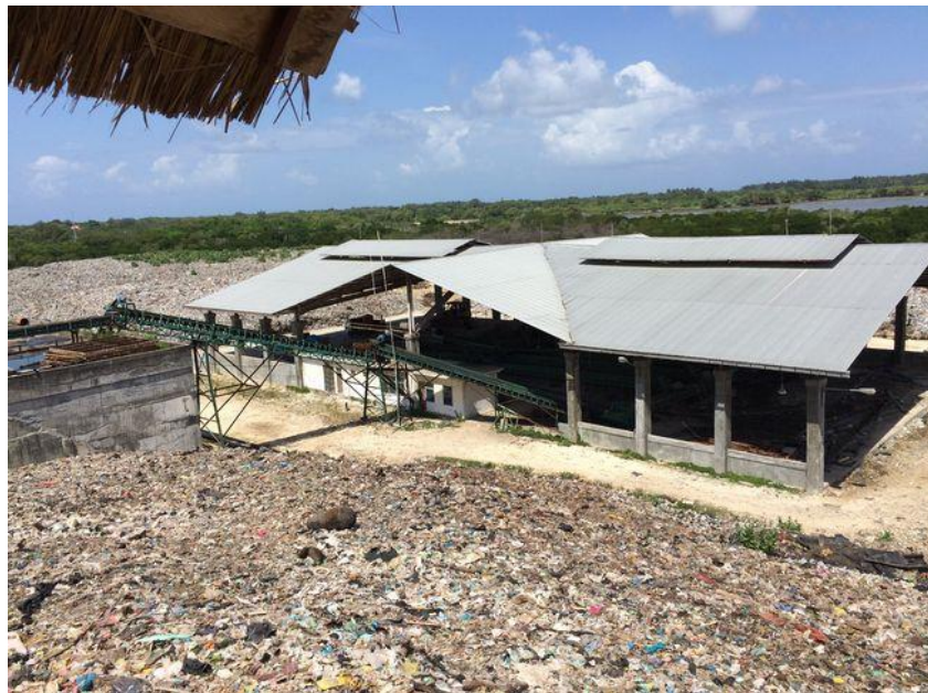
Figure 2.16 NOEI facilities (they are assumed to be the pretreatment facilities for separation)
