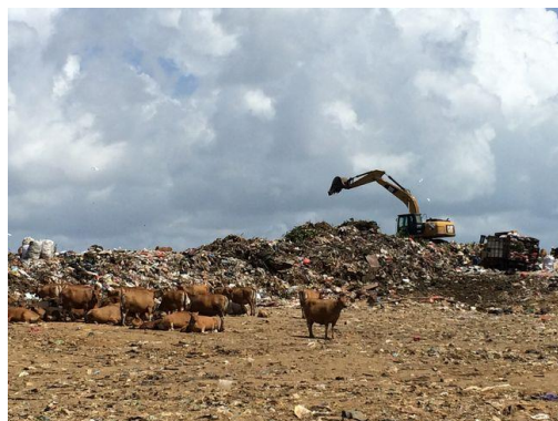
Figure1.2 Current situation of TPA Suwung landfill (As of August 2016)
