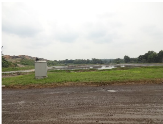
Wastewater treatment reservoir
