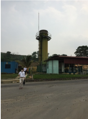
Equipment for burning methane gas collected from the disposal site (the gas engine is currently installed)
