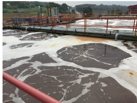
Wastewater treatment tanks (aeration process)
