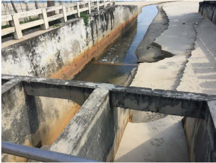
(Photo 4-44. Overflowing wastewater in new city area (2))
