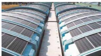
Movable photovoltaic power generator installed over the filter basin in the Kosuzume Purification Plant
