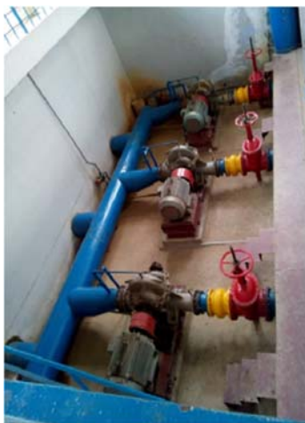
(Photo 4-5. Raw water pump in old Cau Do Level 1 Pumping Station)
