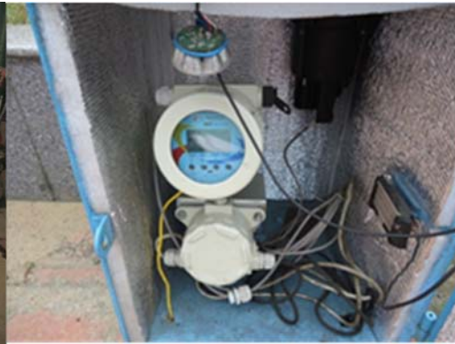
(Photo 4-13. Display of water supply amount in old system)
