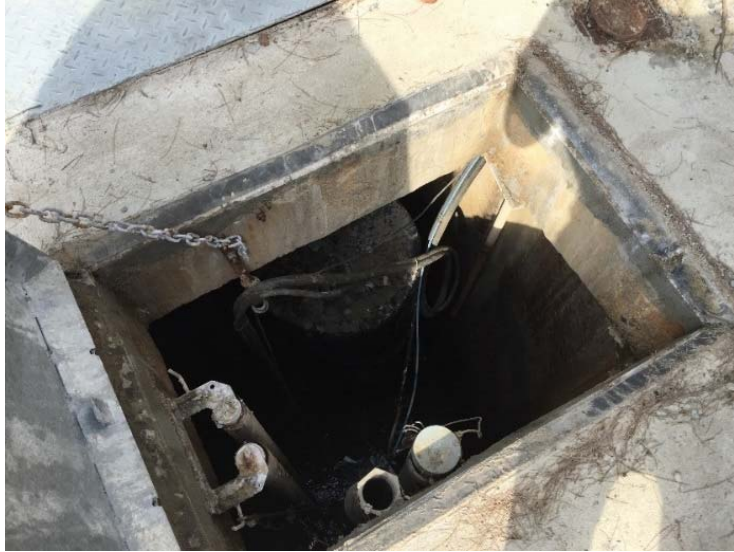
(Photo 4-42. Pump installation location in new city area)
