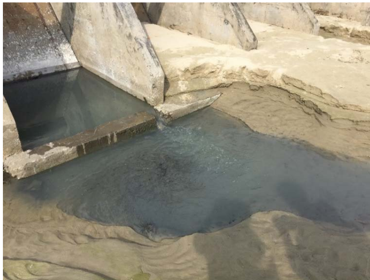
(Photo 4-41. Overflowing wastewater in new city area)
