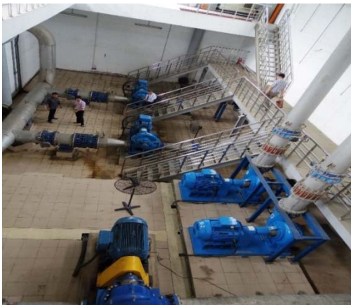
(Photo 4-14. Pumps at new San Bay Level 2)
