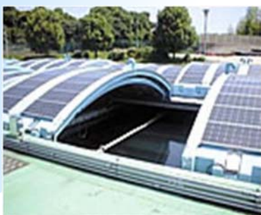
Photovoltaic power generator for the filter basin at the Kosuzume Purification Plant
