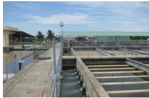
(Photo 4-1. Lamella Sedimentation at Cau Do WTP) (Photo 4-2. Raw water basin for the Cau Do WTP)
