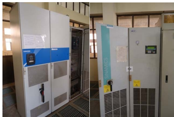
(Photo 4-10. Inverters attached to Cau Do water supply pump)
