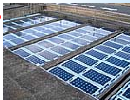
Photovoltaic power generator for the settling basin at the Kosuzume Purification Plant
