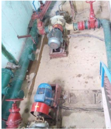
(Photo 4-7. Raw water pump in old San Bay Level 1 Pumping Station)
