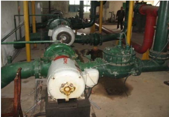
(Picture 4-12. Pumps at old San Bay Level 2)
