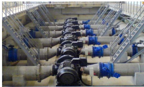
(Photo 4-9. Raw water pumps at Cau Do Level 2 Pumping Station)
