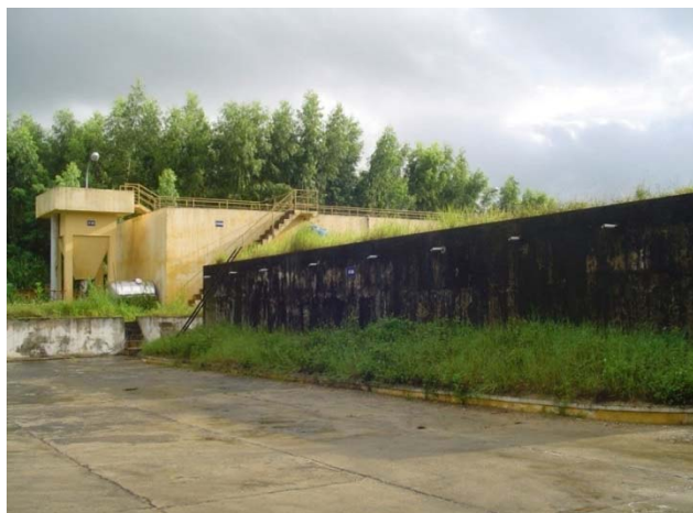
(Photo 4-21. Hai Van water treatment plant)
