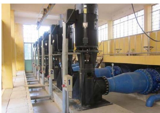
(Photo 4-18. Pumps at An Trach pumping station)
