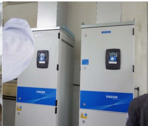
(Photos 4-15. With inverter (VACON Finland))
