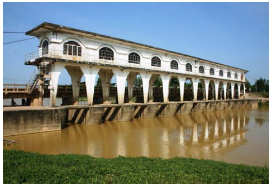
(Photo 4-17. Water intake weir from the Yen River)
