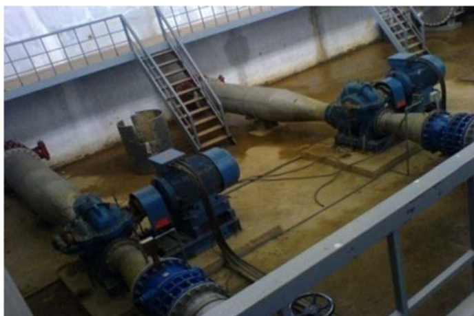
(Photo 4-8. Raw water pump in new San Bay Level 1 Pumping Station)
