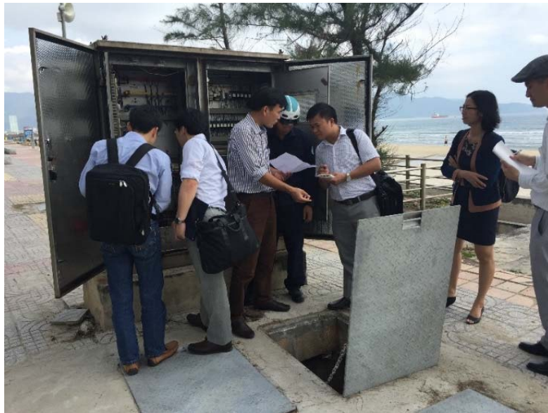
(Photo 4-43. Site visit to pump distribution switchboard)
