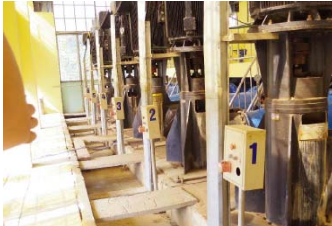
(Photo 4-26. Pumps at An Trach water plant)
