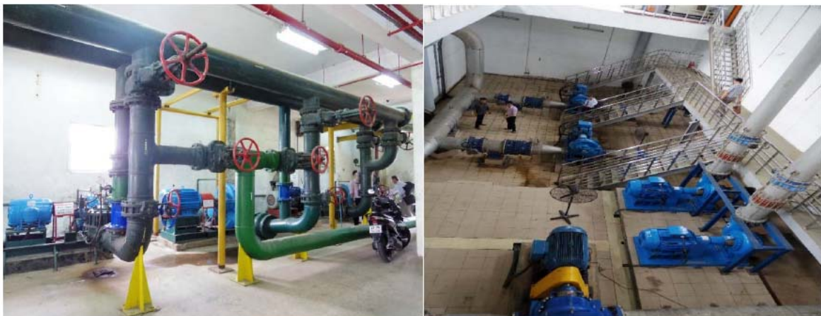
(Photo 4-25. Pumps at San Bay water treatment plant)
