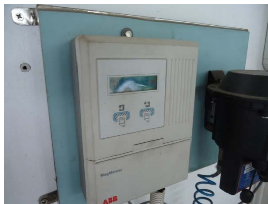
(Photo 4-16. Water supply flow rate display for new system (manufactured by ABB))
