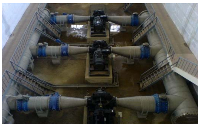
(Photo 4-6. Raw water pumps in the new Cau Do Level 1 Pumping Station)
