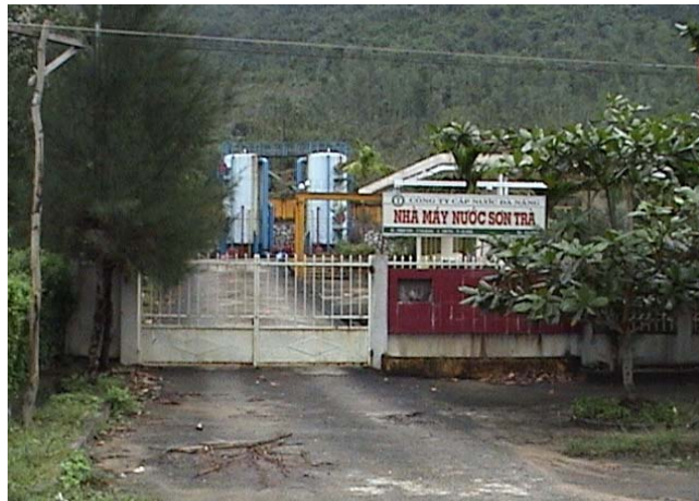
(Photo 4-20. Son Tra water treatment plant)
