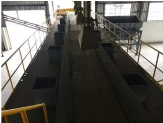
Photo ③ Secondary sorting line (Materials with heavy specific gravity)
