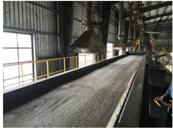
Photo ② Initial sorting line
