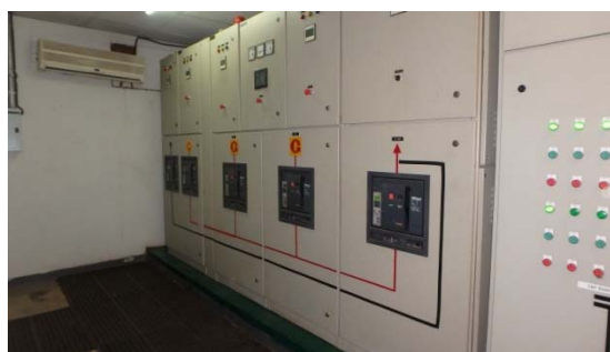
Figure 3-9 : Grid/generator switch board
