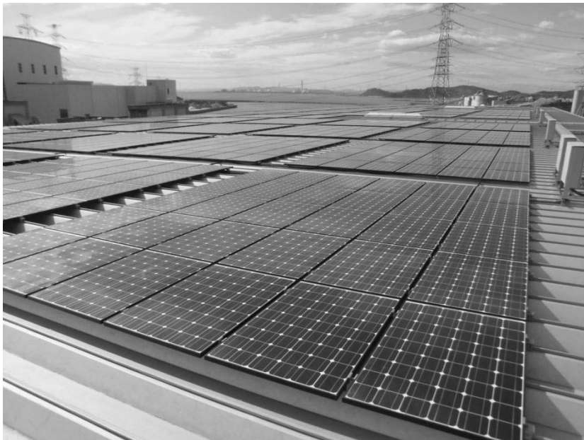
AGC Kansai Factory (Roof Top)
