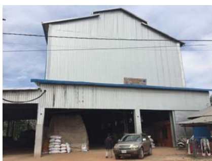
Photo : A rice mill in Siem Reap province
