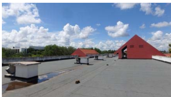
Figure 3-6 : The roof of the main building
