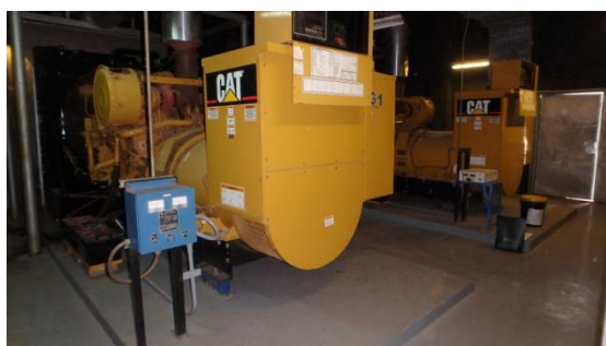
Figure 3-8 : A diesel power generator
