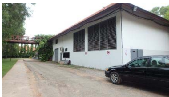
Figure 3-7 : The annex building
