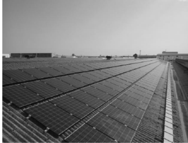
Factory roof after installation
