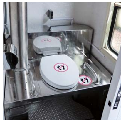
Bio-toilet installed on train car
