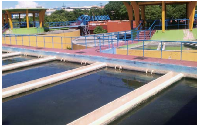
Water treatment facility
