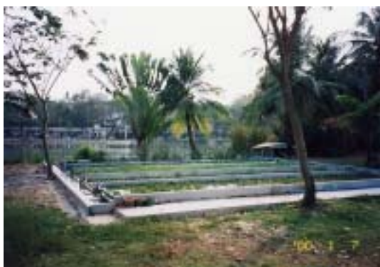
Photo 8-3-1 Bio-park facilities in the Kingdom of Thailand
