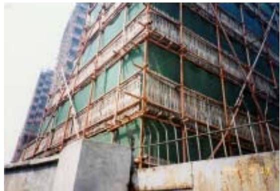
Photo 8-4-8 Use of bamboo at a construction site in China
