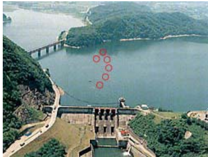
Photo 8-5-2 The position of aeration pipes in Kamafusa dam
