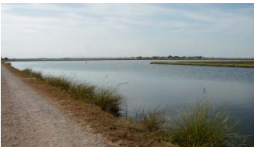
Photo 8-6-1 An oxidation pond at Petchaburi
