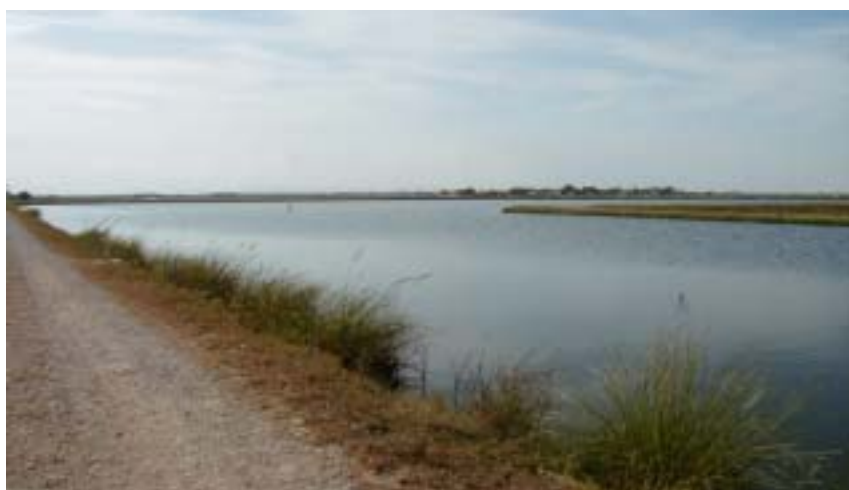
Photo 8-6-1 An oxidation pond at Petchaburi
