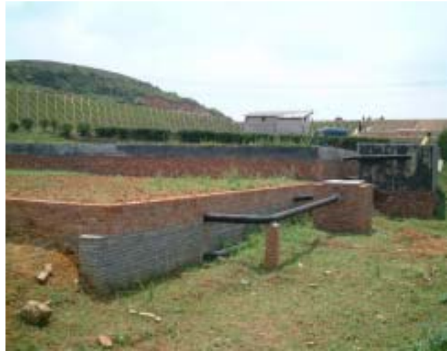
Photo 7-1-6 The soil trench facility constructed by Chinese
